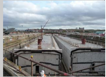
New Submersible sections for the Tunnel
