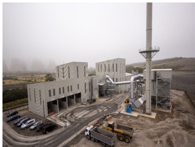
Lightweight Aggregate Plant at Drax
