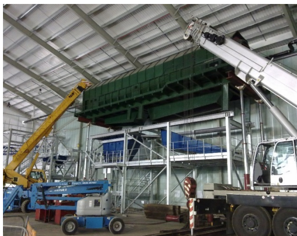
Working at height in an enclosed roof space
