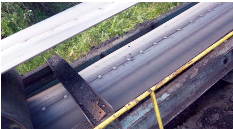
Flexco was able to repair a conveyor tear (above) at Adimitra Baratama Coal's operations using Flexco Bolt Solid Plate 190 fasteners (below).
